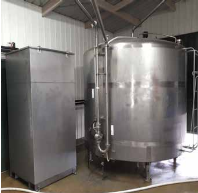
Prototype IES ice-bank system in use in a Waikato dairy shed
